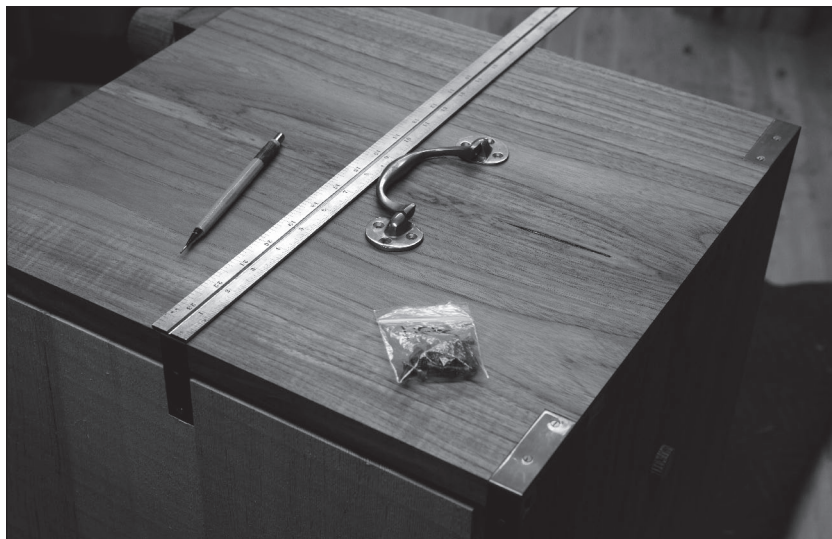
Fig. 4.42 Off-center. Put the lifts slightly above the centerline of each chest component. Here you can see how I aligned the bottom of the lift with the top of the corner brackets. This looks right and works well.
