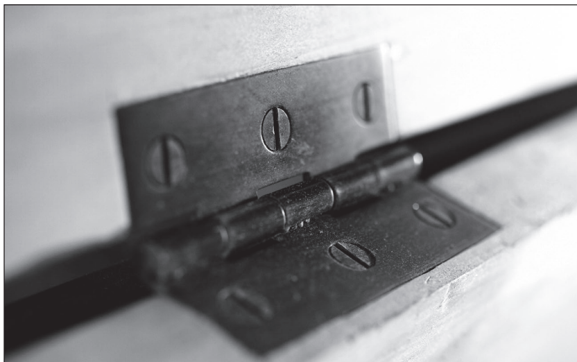
Fig. 3.10 Pretty, standard. Most quality cabinet hinges are extruded these days, though you will still see some that are stamped out then bent. Oh, and there are still blacksmith-made hinges, too.
