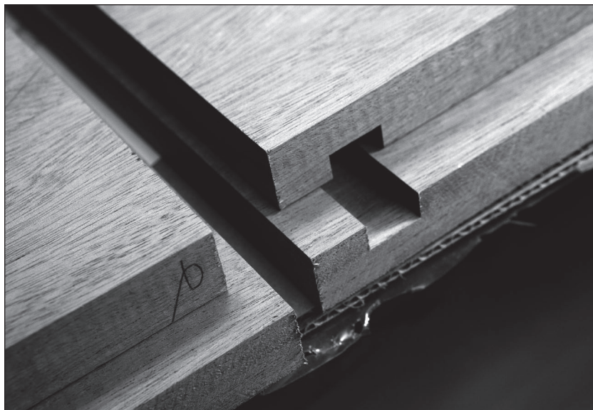
Fig. 10.12 Not in the way. This \frac{3}{4} "-wide x \frac{3}{8} "-deep dado is placed in a spot where it won't interfere with my hinges' screws.
