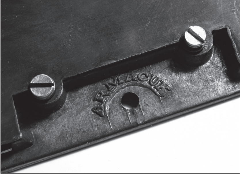
Fig. 3.5 I can read that. Investment casting allows a much higher resolution of detail straight from the mold, such as the manufacturer's name cast onto this pull.
