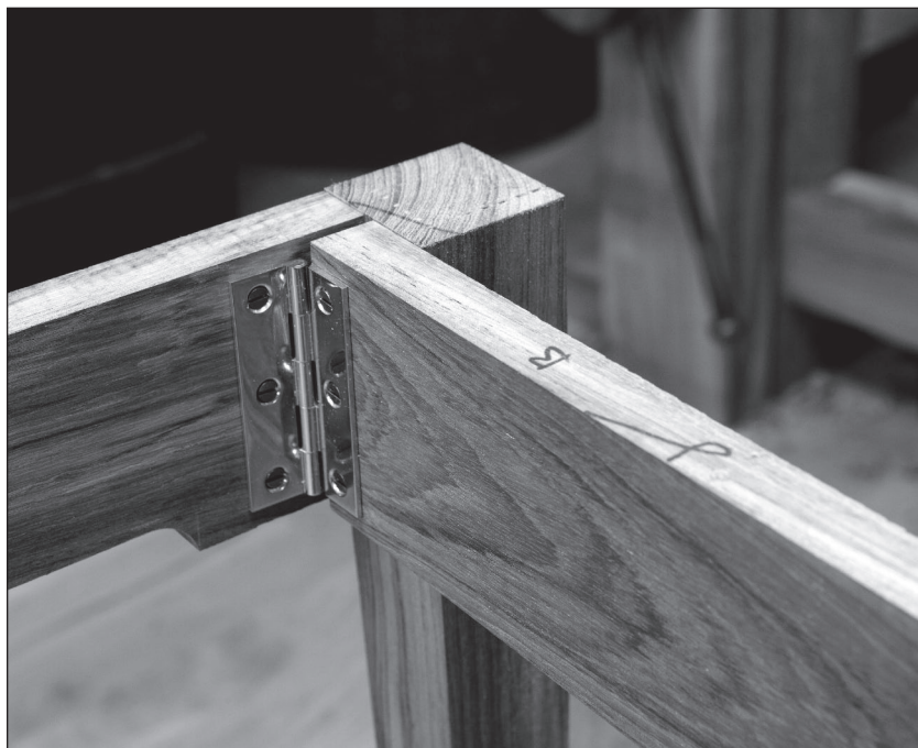
Fig. 9.15 Simple but clever. When the folding apron is connected to the fixed apron, this is what the inside of the table apron should look like.
