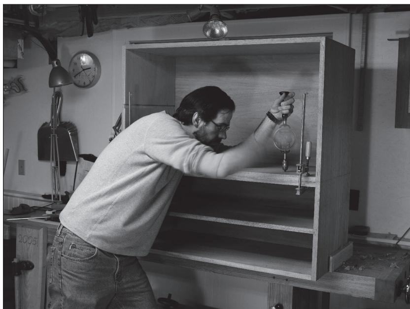
Fig. 4.22 A pilot guides you. With the cases clamped together, drill skinny through-holes into both cases. The pilot will guide the lead screw of the other bits.
