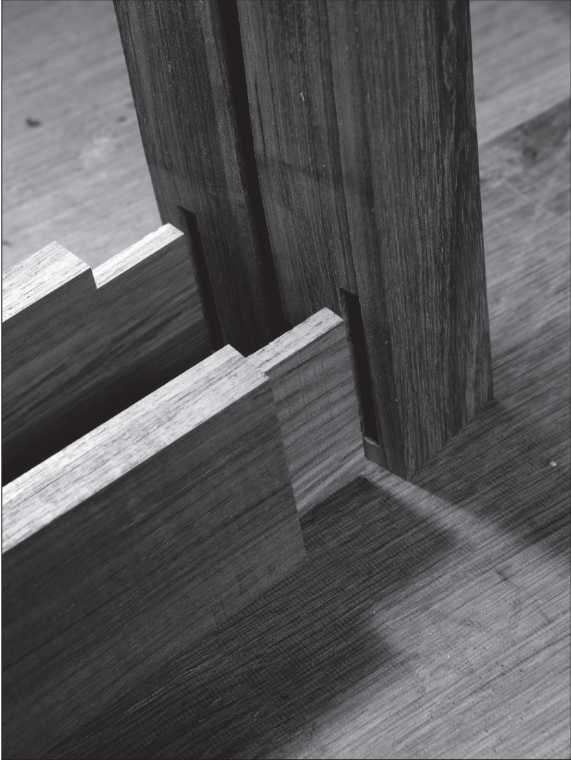
Fig. 9.6 Bareface on the back. Here you can see how there is no face cheek on the inside surface of the apron.
