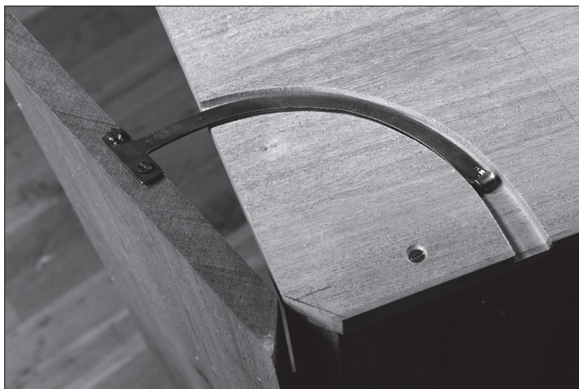
Figs. 5.10 & 5.11 Touchy security. You need quadrant stays to prevent the drop-front from over-extending itself and ripping out your desktop hinges. Careful layout and patterns ensure they will move smoothly through the drawer side. Note that on some secretaries, the drawer side was veneered after the quadrant stays were installed.
