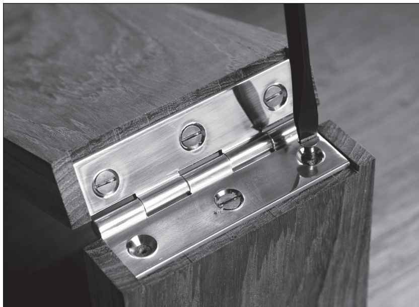
Fig. 9.11 Slotted screws. The appropriate fastener for a piece of furniture from the early 19th century is a slotted brass screw. Modern fasteners (Phillips, Torx, dry-wall etc.) look wrong.
