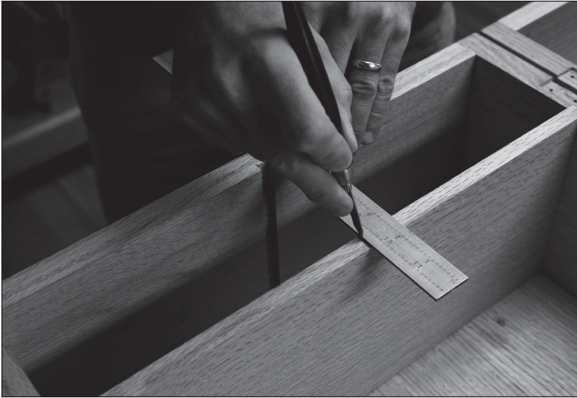
Fig. 11.16 Line up the dados. I cut the dados for the drawer dividers after assembly. Using a square, I lined up the walls of the dados and marked out what needed to be cut away.
