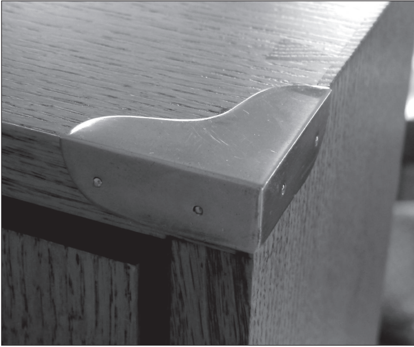
Fig. 3.11 Too easy. Applied corners and brackets are easy to add, and they might seem appealing after so many hours of slaving over the project. Resist. They look fake or cheap.
