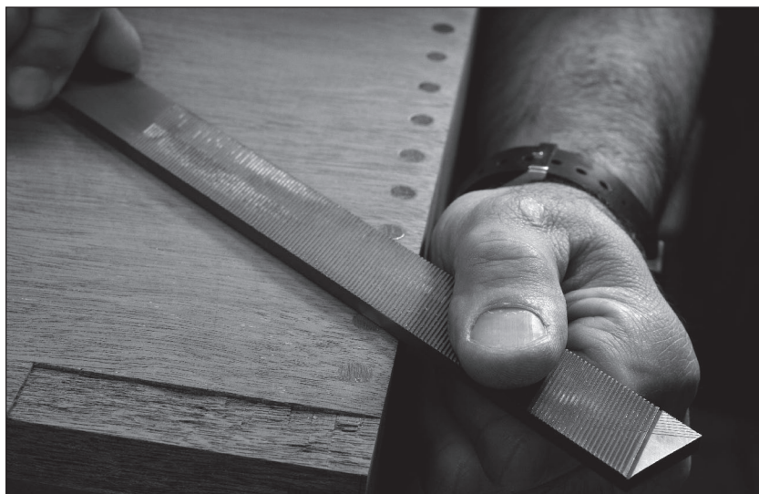
Fig. 8.21 Final filing. The sander will eat away more wood than brass. So after sanding, use a file to level the tops of the screws with a few finishing strokes.
