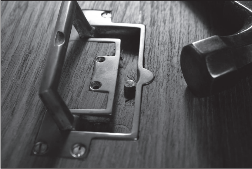
Fig. 3.38 Dowel detail. Depending on the pull, you might need to put a dowel behind the pull to push it forward enough to grab it. It is one of the challenges of inset hardware.
