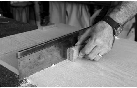
A little crutch. If you lack sawing confidence, you can clamp a batten to the work to help guide your saw. If you are only minorly insecure, a small block of wood pressed against the sawplate can help keep the tool at 0°.
