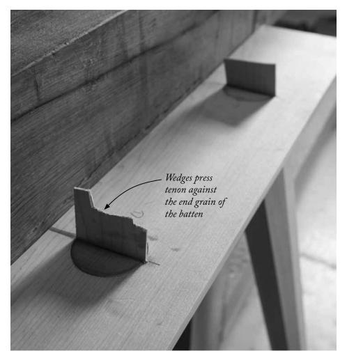
Blind wedges. Glue and wedge the legs into the battens. This locks the legs in place and allows the top to move with the seasons.
