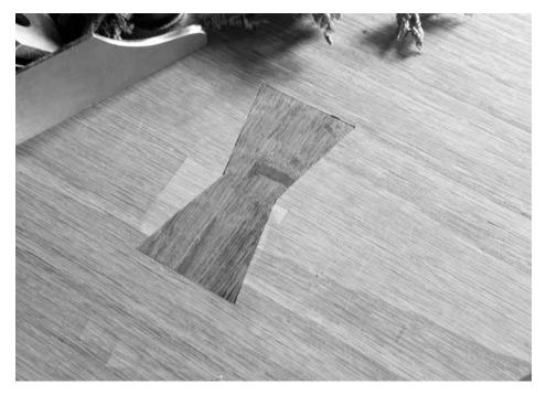
Finished. As you can see, the fit isn't perfect. One knife line got a little rounded over. And a tiny speck of grain popped out. The slab can shift around when you insert the key. However, after some planing, some finish and a little black wax, it will look seamless.
