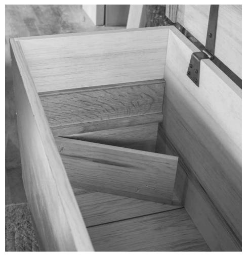
Permanent Jenga. The pine board shown at the bottom puts the lower runner in its correct position. After the first runner is in place, install the second runner on top of it. Then remove the spacer and repeat the process on the other end of the chest.
