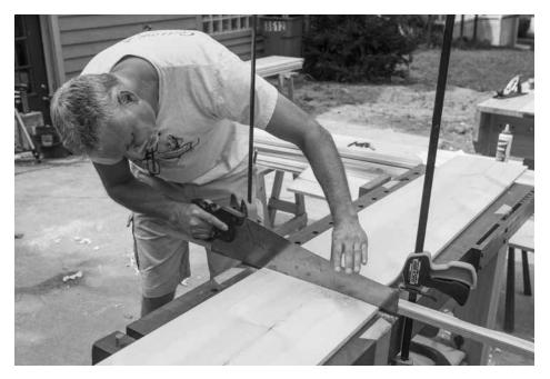
Perfect kerfs. To make sure we got the kerfs right on the first try, we used a fence to guide the saw.
