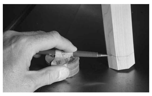
Mark the floor. The pencil point on this 1"-tall block represents the floor. Mark all around the three legs then saw away the waste.
