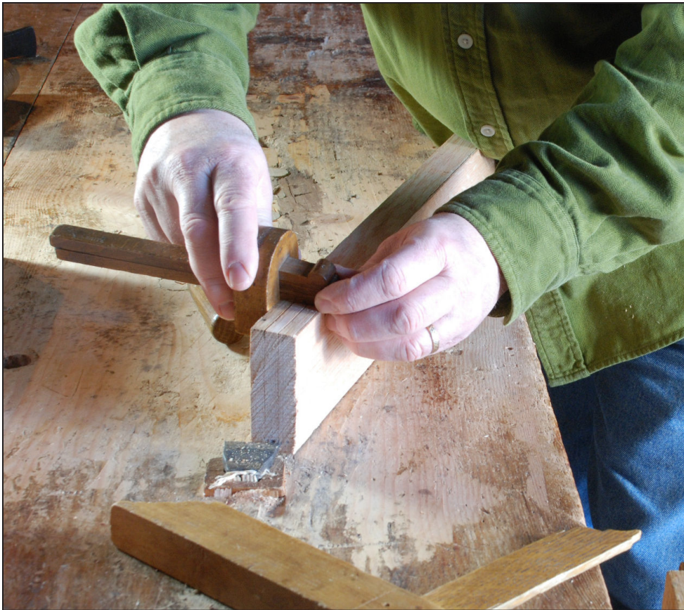
Fig. 4.25 Once again, use both hands to scribe with the mortise gauge. Fix the rail stock in place as well. This reduces any chance of the gauge bumping around. You can shove one end of the stock against the bench hook and the other against your body. Mark all the long sides, then reposition the rail to scribe the end grain.
