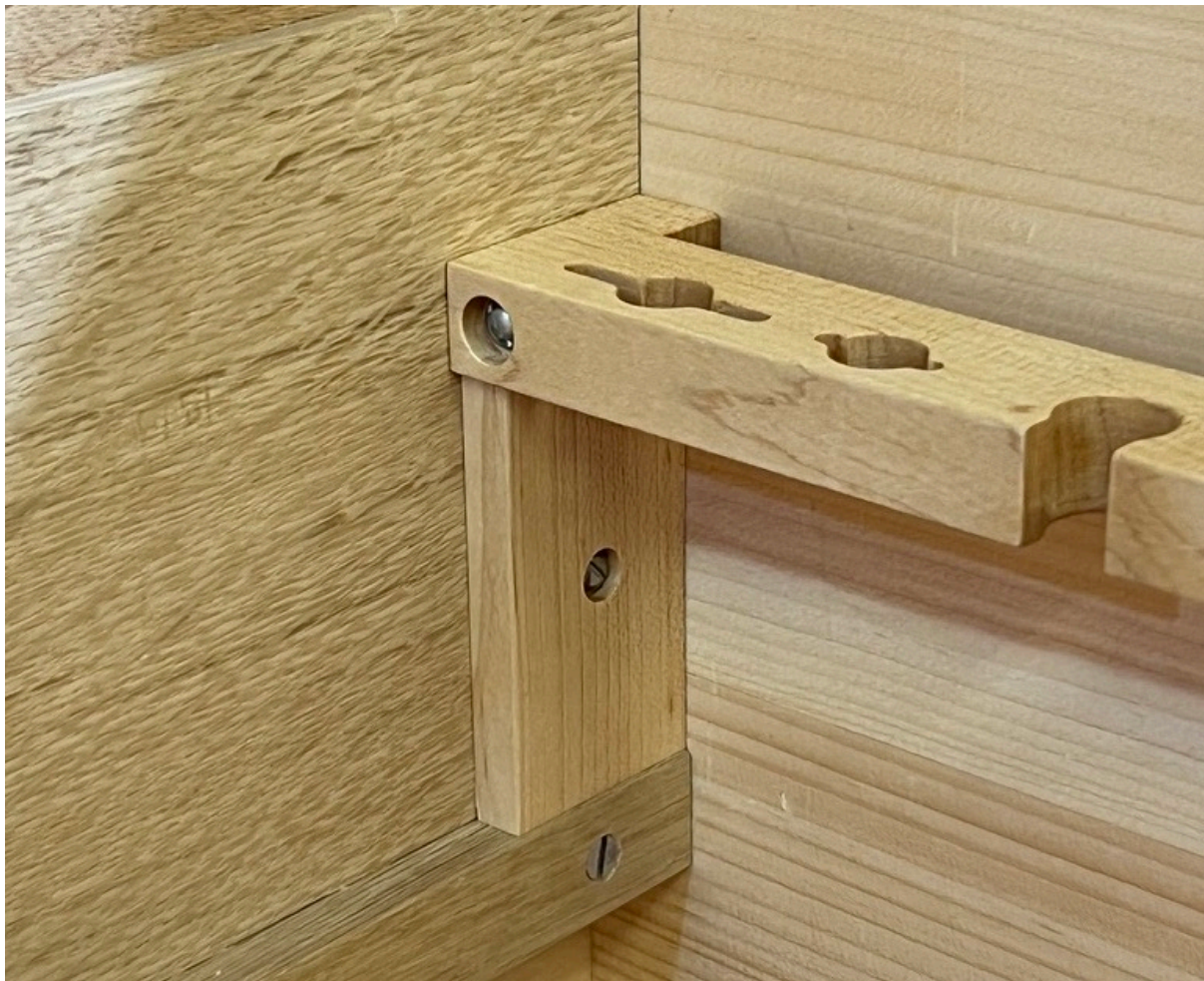
Clearance holes with room for movement.
