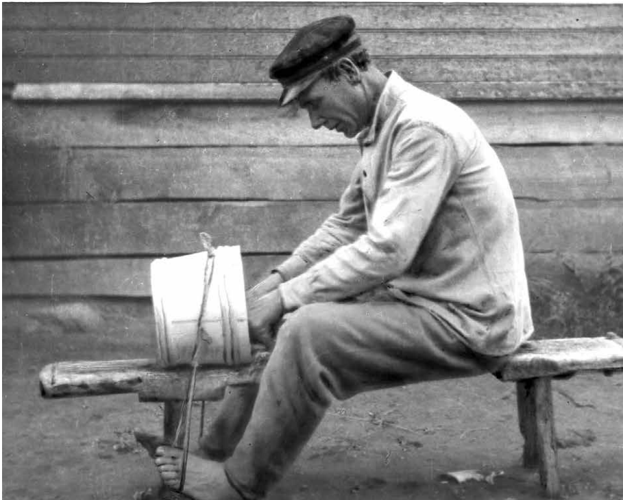
Figure 5.72. Gag order. A rope makes a surprisingly effective hold-down.
