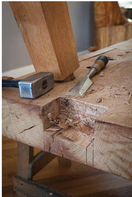
Figure 5.48. Slow going. Chopping out a notch in the end grain is more difficult than performing the same operation in the edge of the benchtop. Saw the sides of the notch. Chop halfway through, then flip the bench and chop the remainder out.
