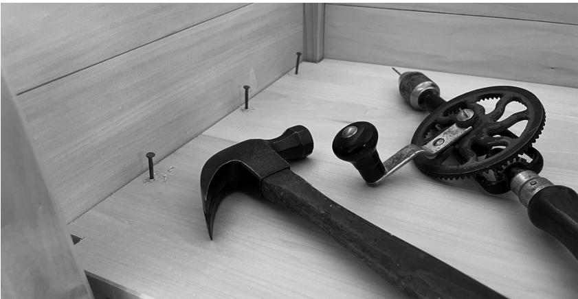
Nailed-in cleats (top) support nailed-in shelves (below).
