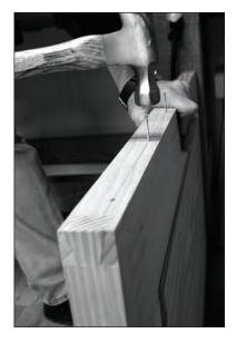
Nails clinch it. Driving cut nails through the skirt and into the lid is a way to ensure that the skirt will remain attached to the lid through heat, moisture and shock.
