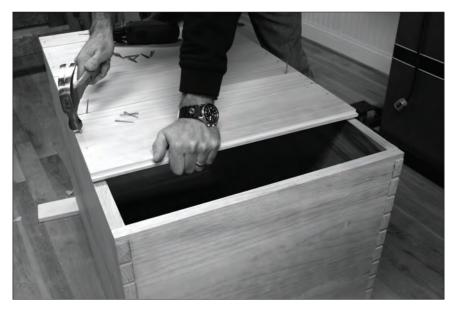
**Nailed to stay.** Cut nails wedge the bottom boards in place better than wire nails ever will. Here you can see that I used the heads of my brads to space the bottom boards. I was out of dimes.
