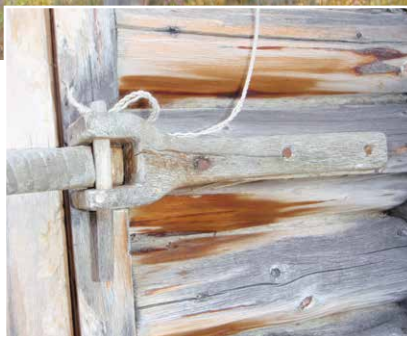
Front of cache. Note the door hinges. (Photo by Monroe Robinson)
