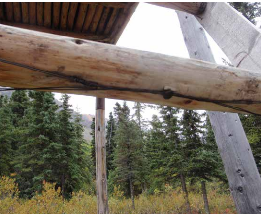
Another two wraps of the wire hold the sides together and act as an emergency support if a rung were to break – lightweight engineering. (Photo by Monroe Robinson)
