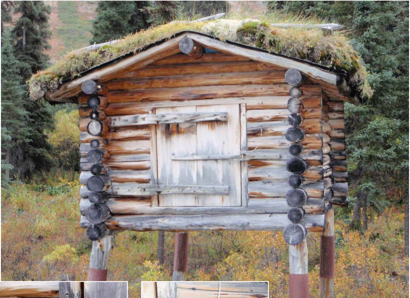
Front of cache. Note the door hinges. (Photo by Monroe Robinson)
