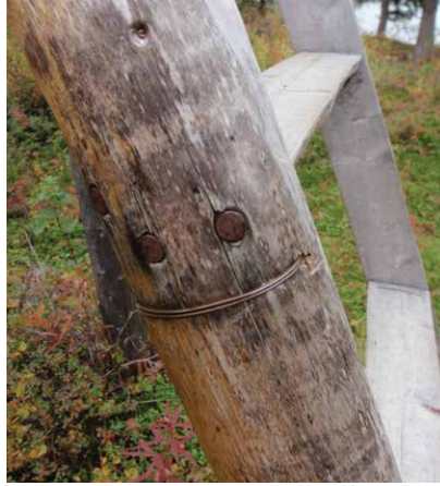
Two spikes hold each end of each rung. (Photo by Monroe Robinson)
