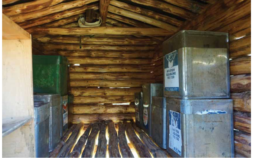
Cache floor stringers, deck poles and 5-gallon storage cans. (Photos by Monroe Robinson)
