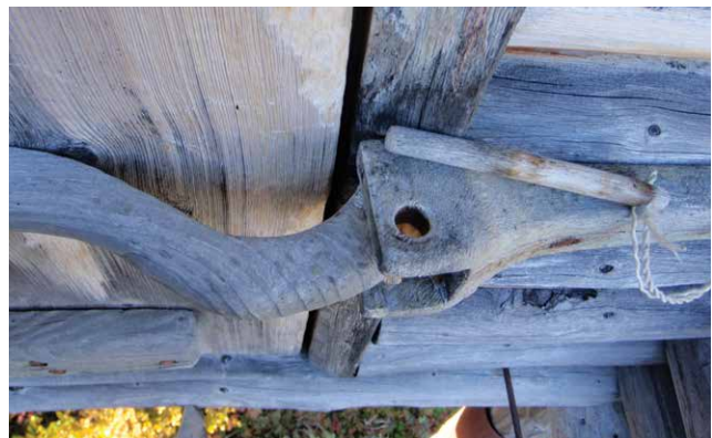
(Left & below) Cache door handle and latch. (Photos by Monroe Robinson)
