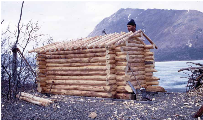
Dick building his cache using his double-bit axe, Greenlee drawknife, the Plumb hatchet, a True Temper hammer and "hurdy gurdy" drill. Note the ice with water along the edge of the lake. (Photos by Dick Proenneke, courtesy of the National Park Service)
