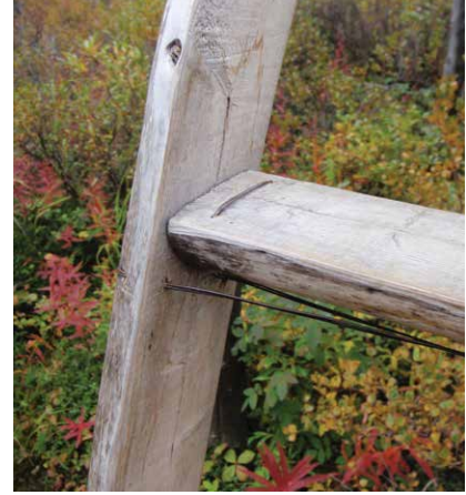
The wire is firmly wrapped two times around the ends of the rungs to help keep the ends from splitting out from the spikes. (Photo by Monroe Robinson)
