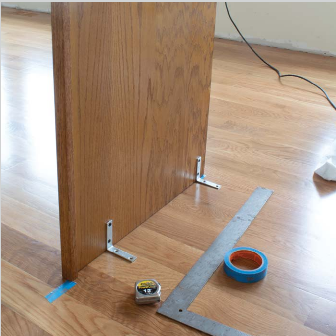
Hidden dishwasher. To make a quick and simple enclosure, I fastened a matching panel to the floor with L brackets, then cut rails to hold the upper end of the panel equidistant from the sink base.
