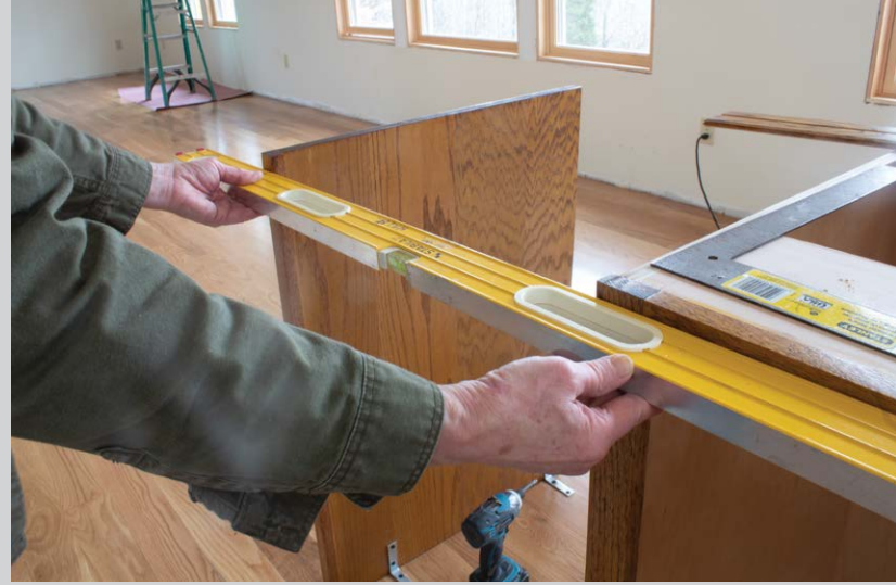
Double check. A straightedge (in this case, a 4-foot level) ensures that the front edge of the panel is in plane with that of the sink base.
