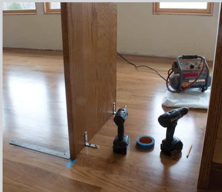
Parallel lines, again. A framing square ensures that the dishwasher panel is square to the flooring.
