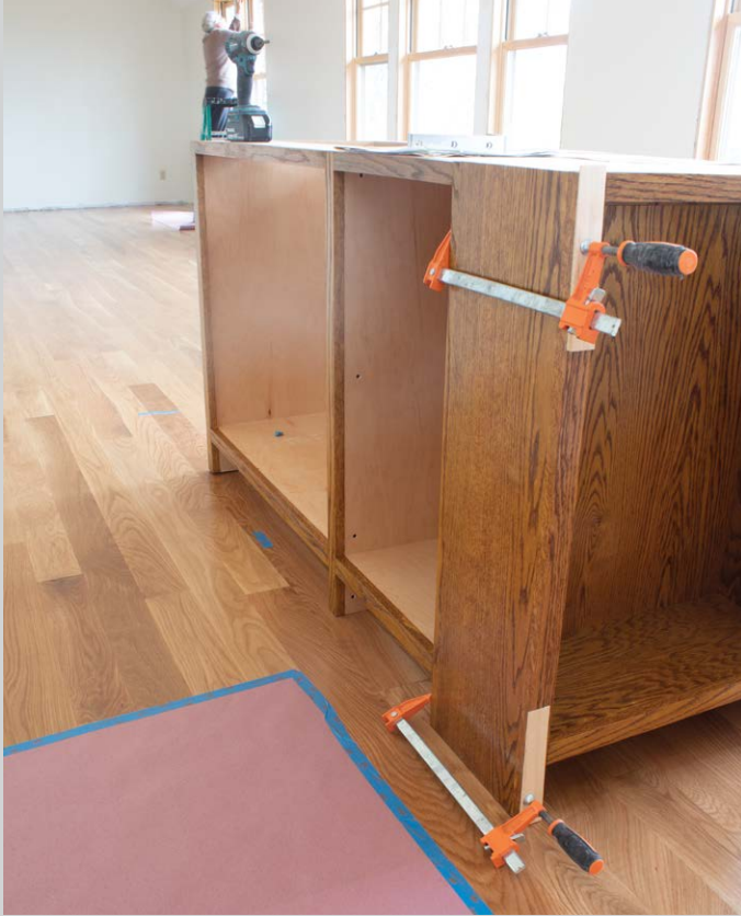
Building blocks. Once the sink base was in, I clamped and screwed the other elements of the island to it.
