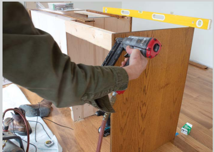
Ready for action. After confirming that all the parts were where they should be, I attached the panel to the sink base at its top.
