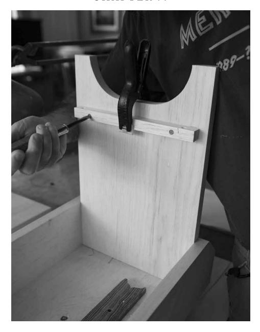
First, secure the cleat. Screw the cleat in place – the clamp helps hold it while you drill the pilot holes.
