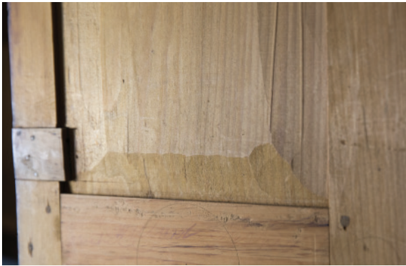
This panel was hastily beveled to fit into the groove of this door.
