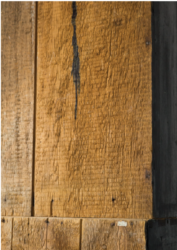
The backs of most of his casepieces are completely unplanned, showing the up-and-down sash saw marks.
