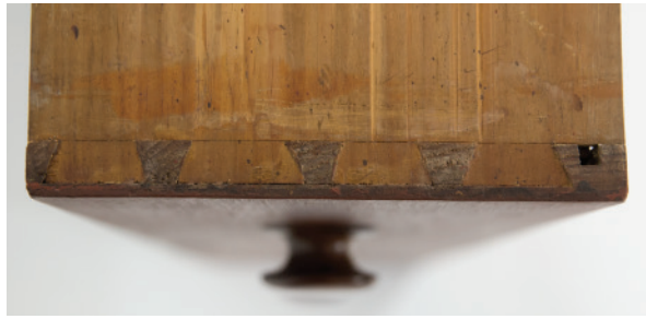
These dovetails, although regular in appearance, all have slightly different angles. This suggests Fisher cut these by eye, without a dovetail maker or template.
