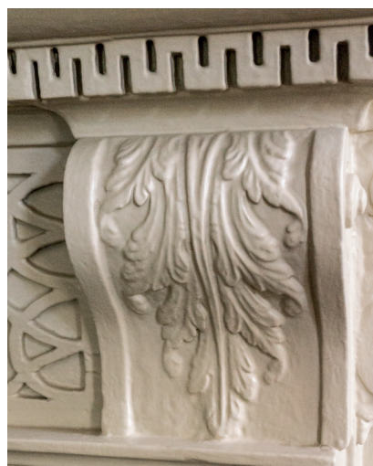
FIG. 4.3 Plaster casting of the hall ceiling medallion, Joseph Manigault House, Charleston, SC. Provided by David Hoffman.
