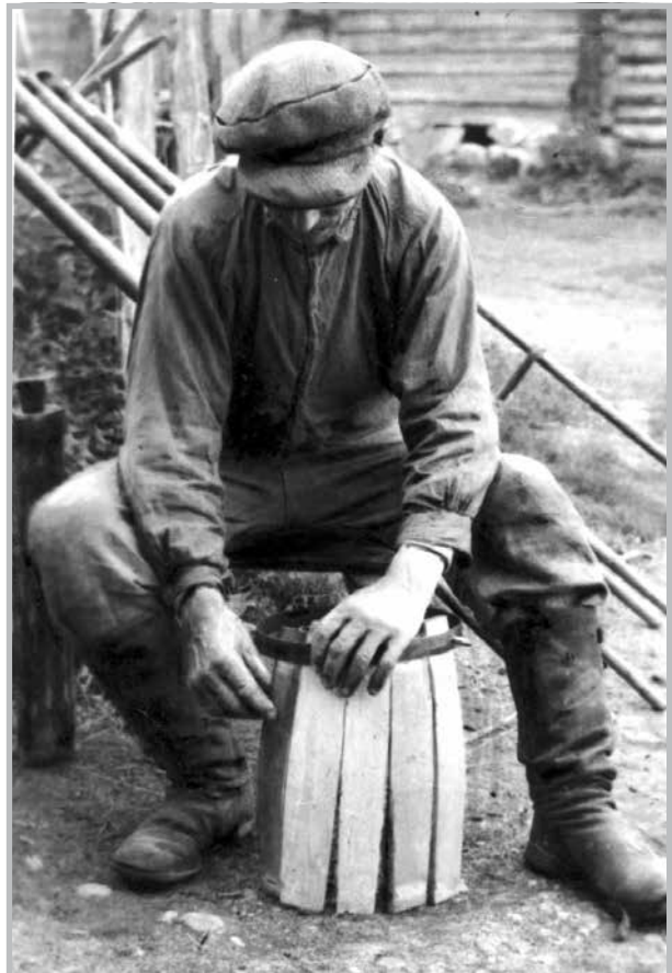
FIG. 113. Assembly of barrel, Avinurme, Vadi village, Photograph by author, 1947. Photo library 1089:74.
