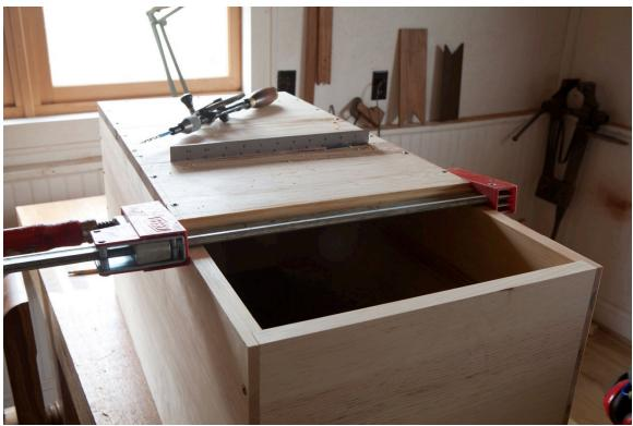
Nails all around. Don't glue the bottom boards, just use nails. I drive three nails into the ends of the carcase. Then I space the nails ever 4" or 5" when nailing into the front and back of the carcase.
