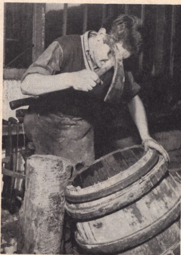
FIG. 4. CUTTING THE CHIME
